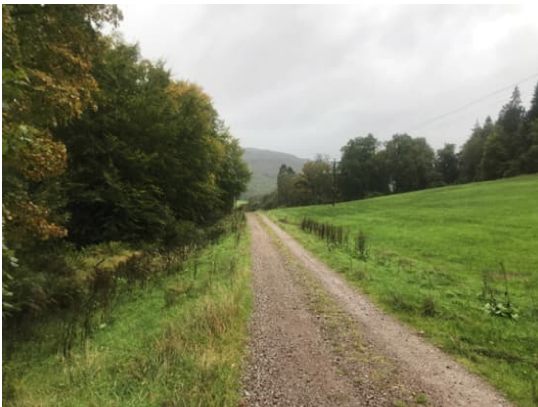
Photograph 46: Section of the existing track, as it passes the foot of Dùn na Cuaiche, which will be temporarily upgraded to serve as a workers access track.
