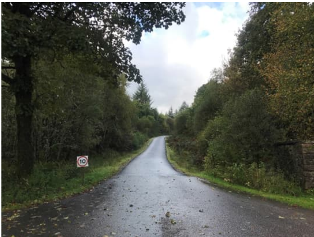
Photograph 48: Section of the existing track near Malt Land which will be temporarily upgraded to serve as a workers access track.
